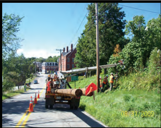
Fairpoint Communications crew relocating utility poles on N. Front St.
